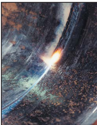
Inside of an 8 in. x .375 in. wall API 5L-X52 pipe, welded in 5G position.
